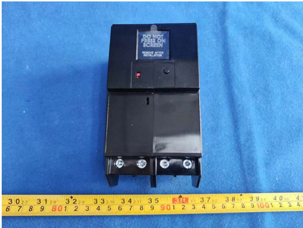
FIGURE 2 240 VAC 60 A WISER CONTROL RELAY (QO260PWX240) BACK APPEARANCE
