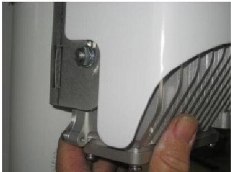
Figure 24 - AirSynergy unit engaged into the bottom slots
