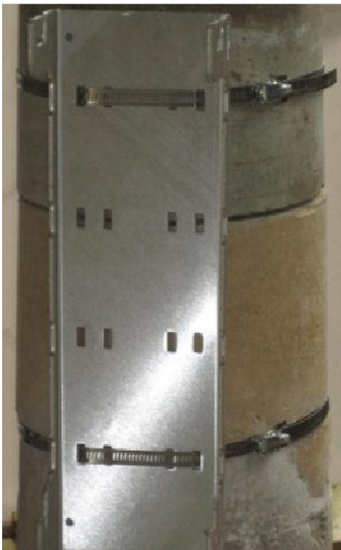
Figure 14 – mounting plate installed on large diameter pole
