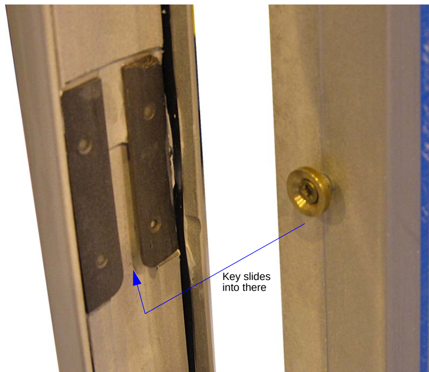
Figure 1.17 Sliding the frame side sections down
