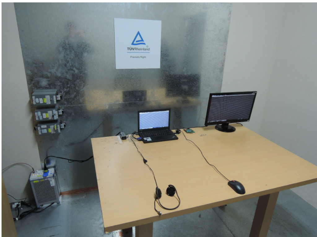
Photograph 6: Set-up for for Mains Conducted testing Front
