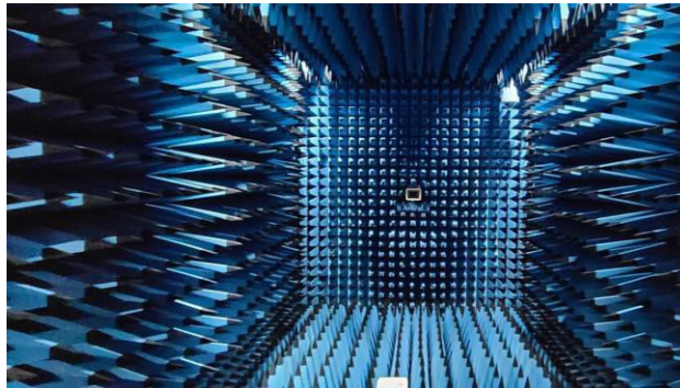
Figure 2: Geometry of Anechoic Chamber for Radiation patterns.
