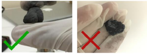
3.2 Roll epoxy into a 2-3 inch strip, then form a ring on the bottom of the Mote mount.
