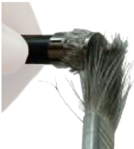
Figure 5-104 Clearing impurities
