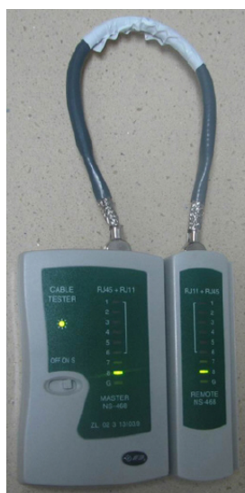
Figure 5-86 Testing the conduction and connections of wires
