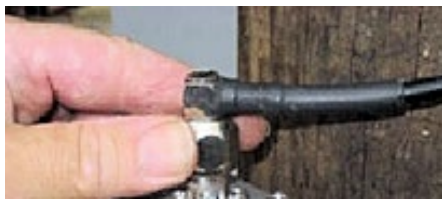
Figure 10: Connecting Antenna RF Cable
