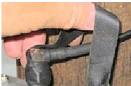
Figure 11: Weather-proof the Connection
