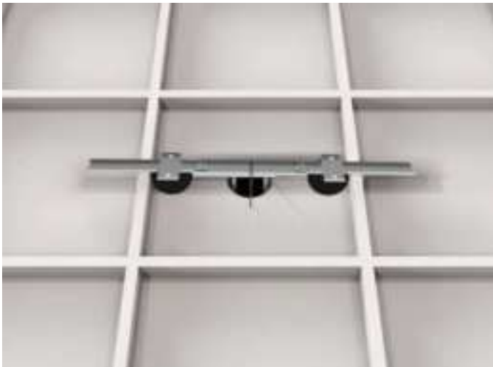
Figure 65. Placing the Bracket I & VI 2
