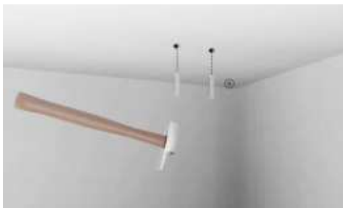
Figure 50. Insert Plastic Wall Plugs
