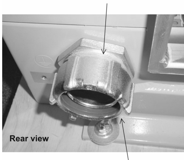
2" FLEXIBLE CONDUIT FITTING (CUSTOMER PROVIDED)
