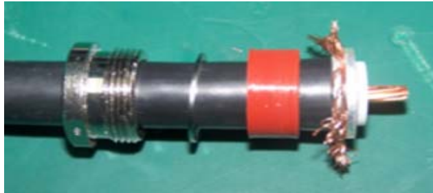
FIGURE 76 - INSERTING INSULATING PLATE
