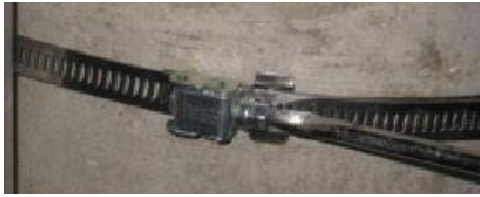
Figure 13: Tighten clamp bands
