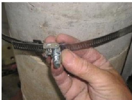
Figure 11: Assemble clamp bands (4 required)
