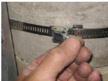
Figure 12: Press down locking mechanism
