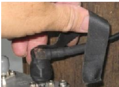
Figure 8: Weather-proof the connection
