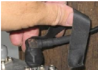
Figure 33: Weather-proof the connection
