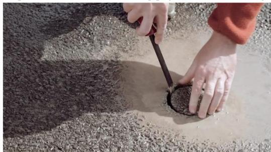
Step 6: Level sensor in hole using a base of sand.
