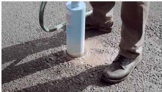
Step 5: Remove core, using pry bar if necessary.
