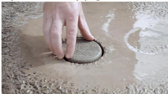
Step 8: Seal sensor in place.
