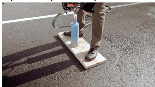
Step 4: Finish drilling hole (4" diameter x 3" deep).
