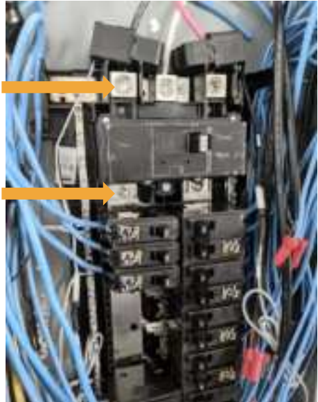
Figure C – Typical Main Breaker Electrical Panel
