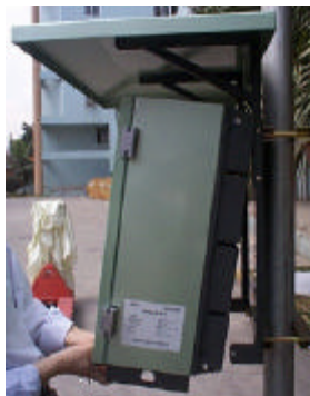
FIGURE 9 PUSHING CHASSIS INTO POSITION-POLE MOUNTING
