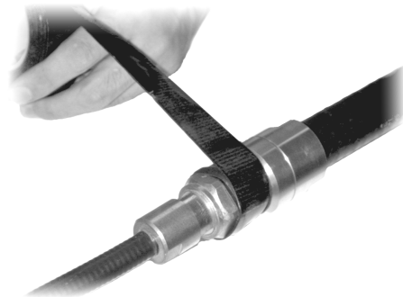
FIGURE 48 WATERPROOF ADHESIVE TAPE WRAPPING (1)
