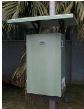
FIGURE 11 MOUNTED CHASSIS-POLE MOUNTING
