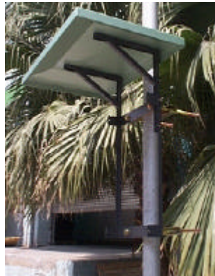
FIGURE 7 SUNSHADE INSTALLED -POLE MOUNTING
