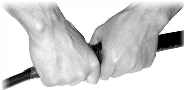
FIGURE 50 WATERPROOF ADHESIVE TAPE WRAPPING (3)
