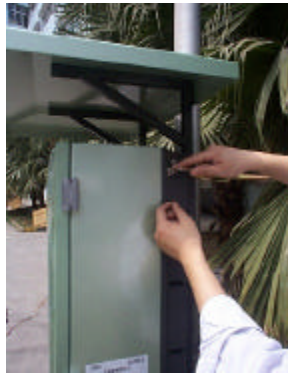
FIGURE 10 FASTENING THE CHASSIS BODY -POLE MOUNTING
