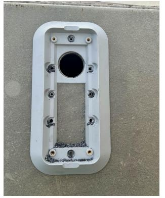
8. Using the rivet tool, set the 8 rivets in the holes.
