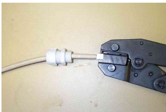
Step 4: Insert conductors and crimp
