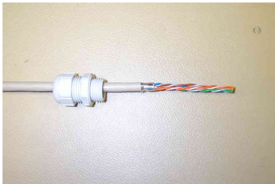
Step 2: Strip the outer insulation
