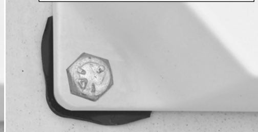
Gasket Compression Level Not Recommended
