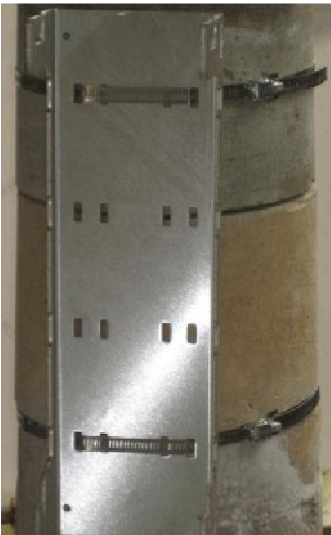
Figure 14 – mounting plate installed on large diameter pole
