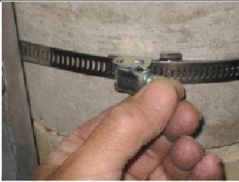
Figure 12 – press down locking mechanism
