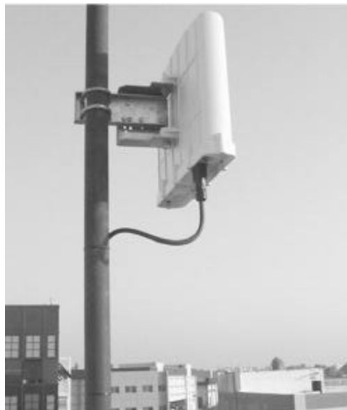
Figure 4-1: Typical BSR Installation
