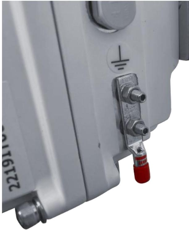
3. Strip the 8 AWG Ground Wire as necessary, insert into wire barrel of Grounding Lug, and double crimp using appropriate tooling.
