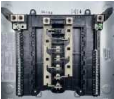
Figure B – Typical Main-Lug-Only Electrical Panel Busing
