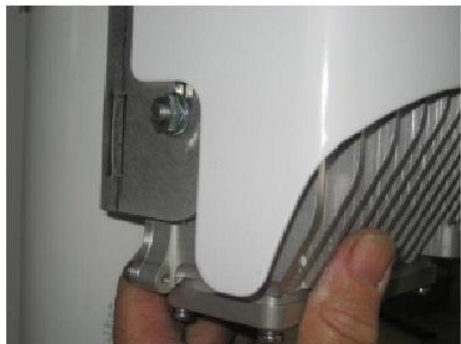
Figure 24 - AirSynergy unit engaged into the bottom slots
