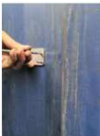
Figure 2-6a Fixation of Mounting Bracket
