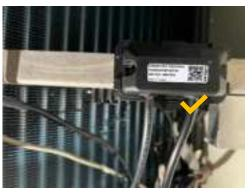
16. Disconnect the humidity sensor from the communication cable and connect the transceiver to the communication cable and the humidity sensor.
