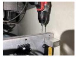
14. Use a screwdriver and 2 screws to mount the bracket.
