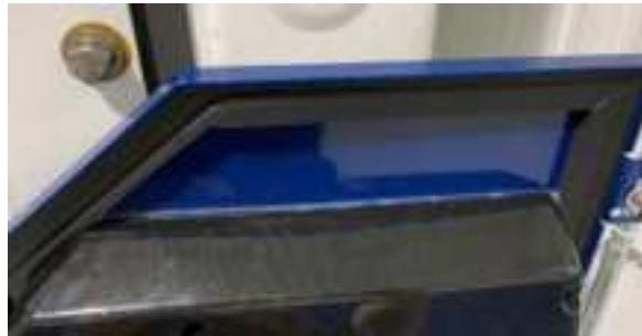
Figure 7b: Caulking of Rain Shield
