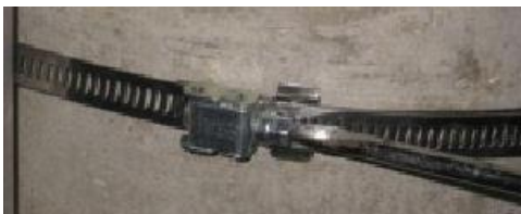
Figure 13 – tighten clamp bands
