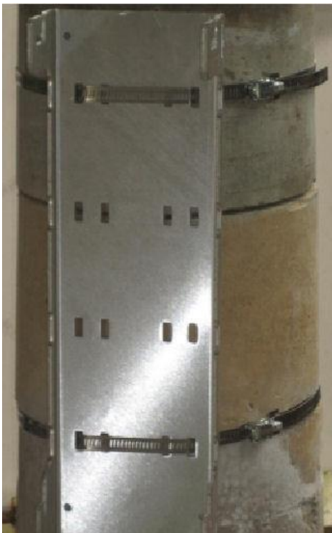
Figure 14 – mounting plate installed on large diameter pole
