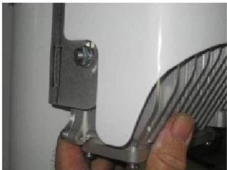
Figure 24 - AirSynergy unit engaged into the bottom slots
