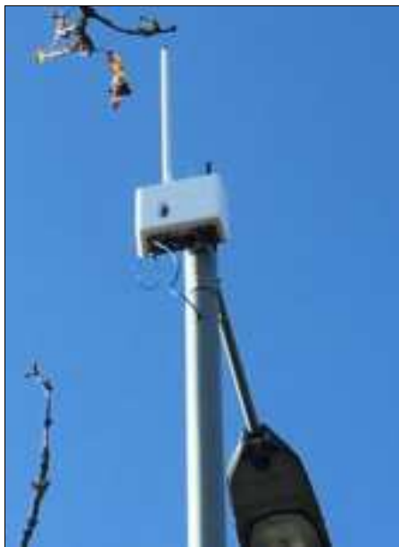
Strap-mount Basestation installation showing power cable connection
