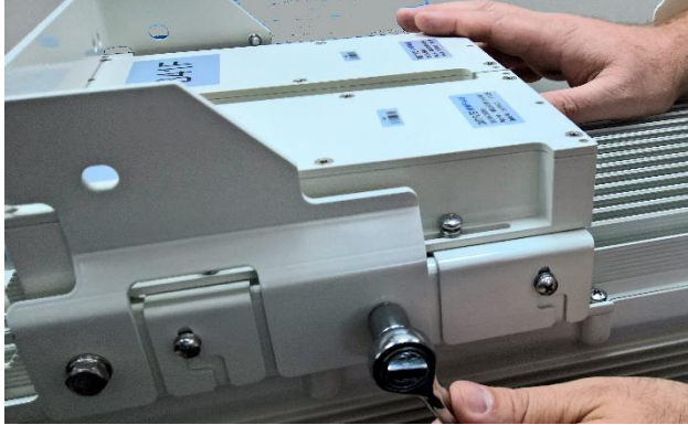
Figure 12: Tighten Hex Head Bolts
