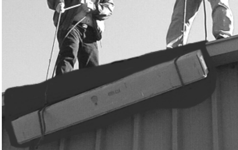
Figure 3-2 Hoisting materials to the installation location
