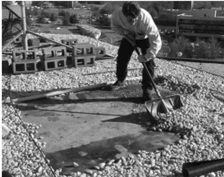
Figure 3-3 Clearing gravel from the installation location
