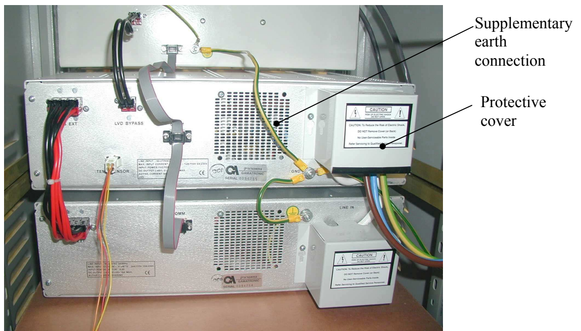
Figure 7-15: Fitting protective covers over terminal block
