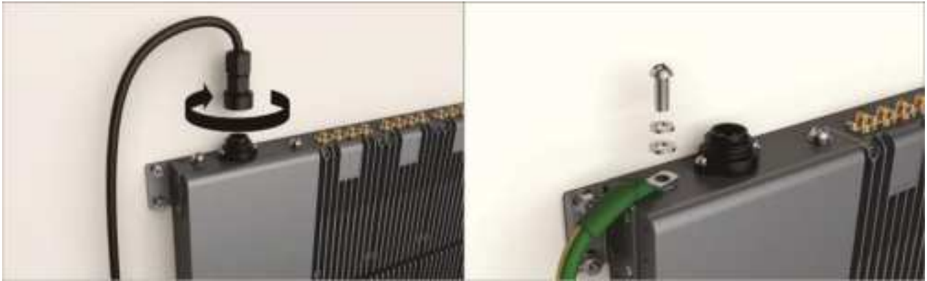
Figure 12. Connect Power and Ground Cables
